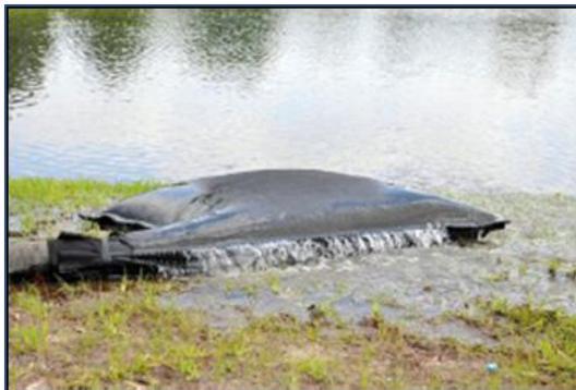
Plate 3-1 Silt Bag with water being pumped through.
