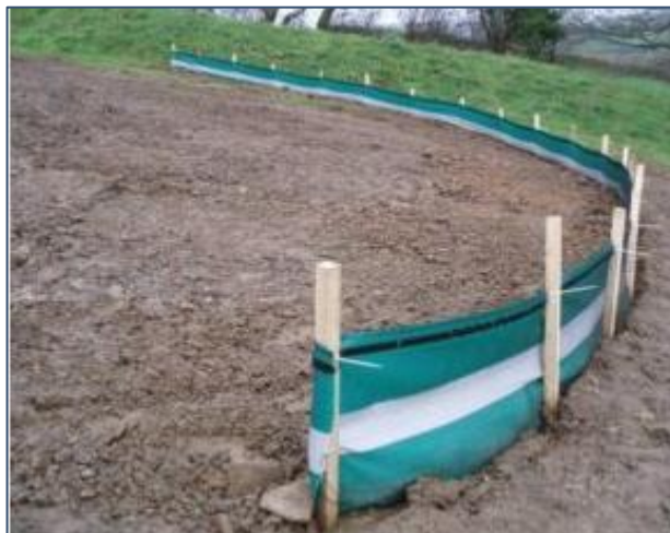
Plate 3-4 Embedded Silt Fence
